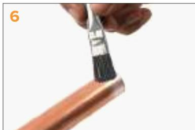
Immediately after cleaning, apply flux to the mating surfaces. (Fig. 6)
