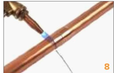
Add the filler rod to the mouth of the fitting, allowing the brazing alloy to melt and flow into the annular gap. (Fig. 8)
