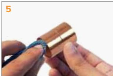
Clean the socket of the fitting with a brush or wire wool. (Fig. 5)
