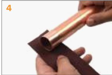
Clean the end of the tube with a cleaning pad or wire wool. Ensure all oil, grease, and heavy oxides are removed. (Fig. 4)
