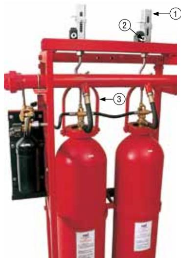
This device is used to automatically monitor the contents of the CO2 cylinder. When the CO2 gas falls the indicator on the device will show that it is empty and an optional Micro-switch can be installed to send a signal to the control panel. This is the most effective method of monitoring the CO2 gas in the cylinders.
