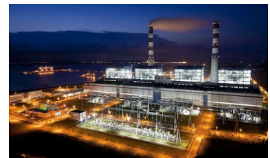
Hangzhou Power Plant of Banqiao Group
